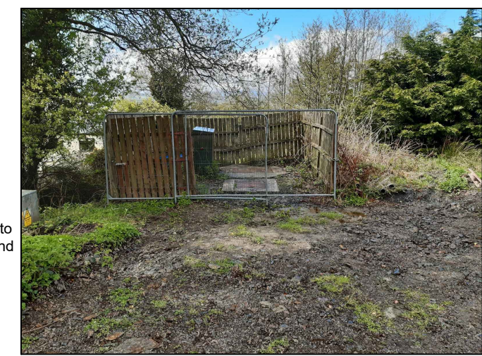
Existing Pump Station to be Decommissioned and Demolished
